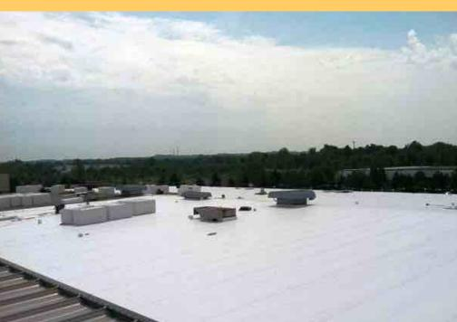
The leading roof membrane is Single Ply roofing, a superb choice for retail, commercial and flat roofs. Single Ply roofing consists of rubber polymers made from prefabricated sheets of material. Preferred offers a complete line of white and colored single ply roofing membranes.
