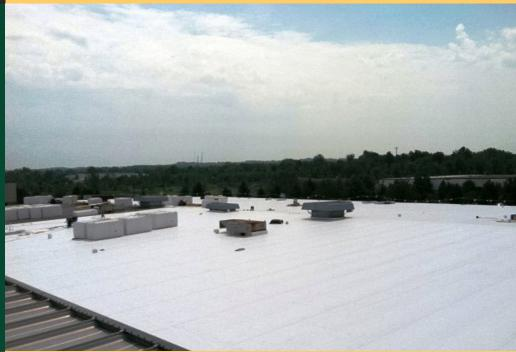
The leading roof membrane is Single Ply roofing, a superb choice for retail, commercial and flat roofs. Single Ply roofing consists of rubber polymers made from prefabricated sheets of material. Preferred offers a complete line of white and colored single ply roofing membranes.
